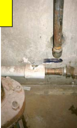
Riser Room Water Shutoff
